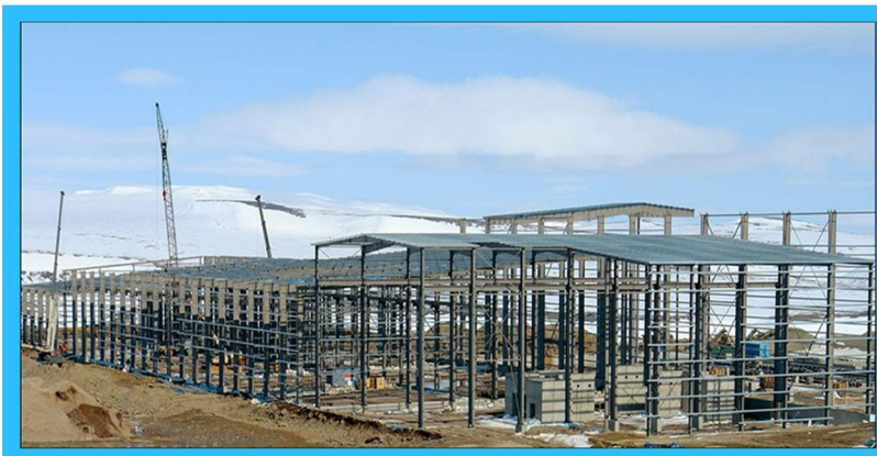
Kinross Gold Kupol Gold All Process Buildings, Truck Shop & Recreation Building
