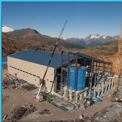
Pretivm Brucejack Gold Mine Mill Building
