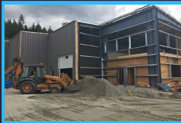
Kanaka Business Park Burnaby Saw Manufacturing
