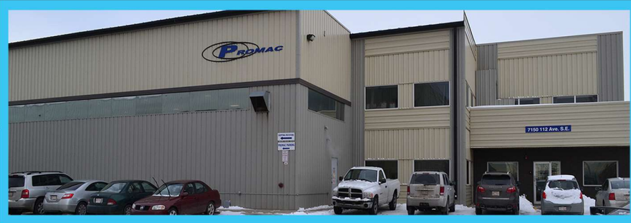
Promac Industries Office & Manufacturing Buildings
