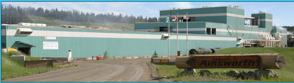
Ainsworth (Norbord) 100 Mile House All OSB Plant Buildings
