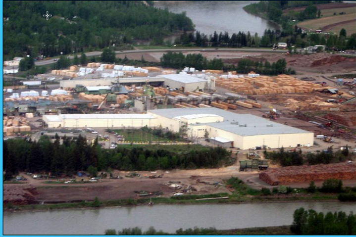
West Fraser Quesnel Sawmill, Saw Gallery, Sorter/Stacker & Warehouse Buildings
