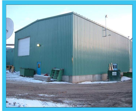
Canfor Radium Planer Mill Building
