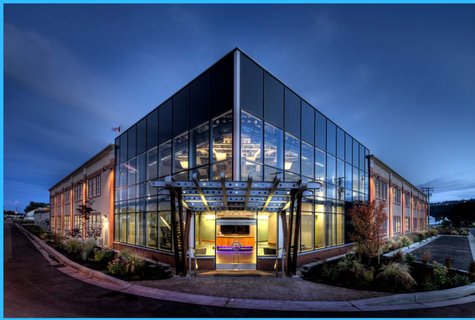
Viking Air- Sydney, BC Manufacturing and Maintenance Facility
