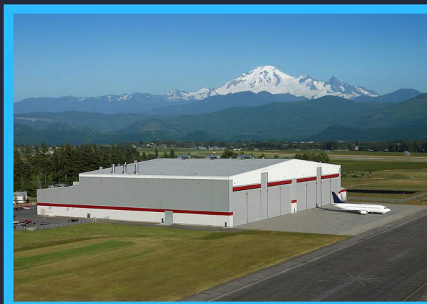
Cascade Aerospace- Abbotsford, BC Maintenance Hangar
