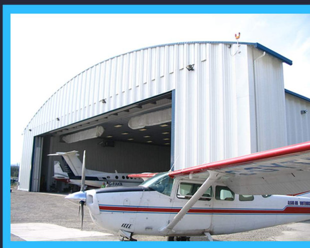
Alkan Air- Nanaimo, BC Airplane Hangar & Hangar Door Addition
